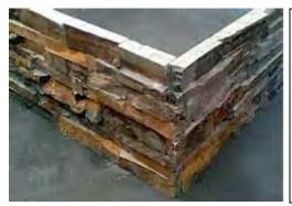
Use of non-historic artificial man-made concrete stone products designed to emulate stacked stone or other historic stone materials are not appropriate and are discouraged.
