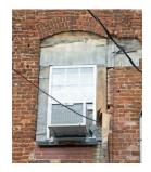
Example of window AC unit inappropriately installed on front façade resulting in replacement and alteration of original window framing.
