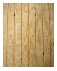
Modern 4 foot by 8 foot T-111 exterior siding panels is inappropriate for exterior repairs or additions.
