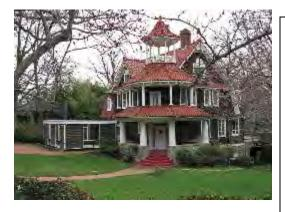
An example of an inappropriate addition. Addition on left is not compatible with the original structure in massing, roof shape, window design and pattern and does not coordinate with the style and features of the original structure.
