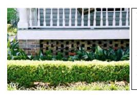
The use of wood or brick lattice design is more desirable than using solid materials for foundation infill to provide proper ventilation and to preserve the historic character of the building.
