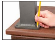
Mark and Pre-drill Holes
