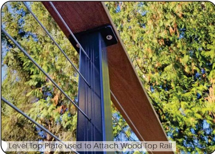
Level Top Plate used to Attach Wood Top Rail
