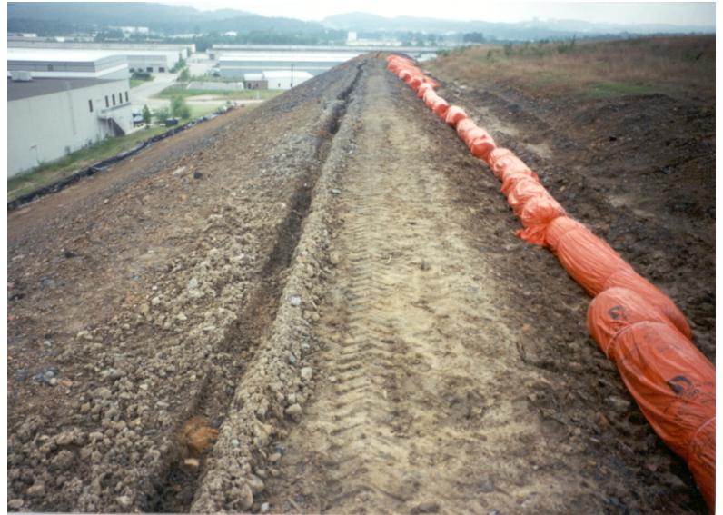
Step Three—Prepare the anchor trench.
