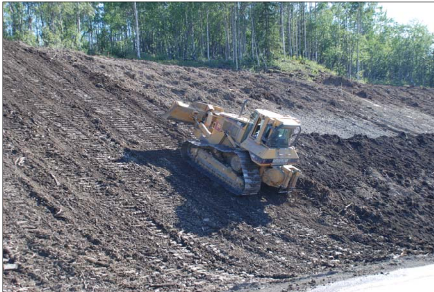
Figure 2: Embankment and Fill Areas Should be Rolled with a Crimping or Punching Type Roller or Track Walked so that Track / Cleat Marks from the Equipment Form an Indentation on the Slope that is Parallel to the Contour of the Slope (Perpendicular to the Flow of Water Moving Down the Slope).
