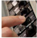
All Panel Breakers and Main Breaker will be placed in the off position. (By the electrical provider APS/SRP). Builder to turn on breaker and verify temporary power outlets functioning prior to Lock-out / Tag-out.
