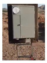
It is extremely important to inform and educate onsite workforces about the hazards of energized Electrical Panels. The panel will be placed in its permanent position long before the house is built. The panel will be supported by 2 metal legs. These legs will remain in place and be out of sight once the house is nearing completion.
