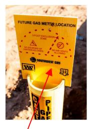
No Gas Line installed (Sleeve Only) Gas Line & Sleeve Installed Gas Clearance Zone
