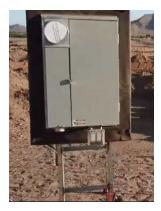
It is extremely important to inform and educate onsite workforces about the hazards of energized Electrical Panels. The panel will be placed in its permanent position long before the house is built. The panel will be supported by 2 metal legs. These legs will remain in place and be out of sight once the house is nearing completion.
