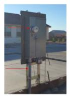
**Recognize the Hazard:** Meter and Riser installed, an Electrical Hazard exists!
