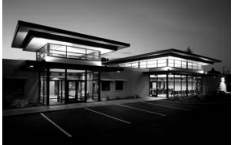
The Inland Northwest AGC building after its 2002 renovation.
