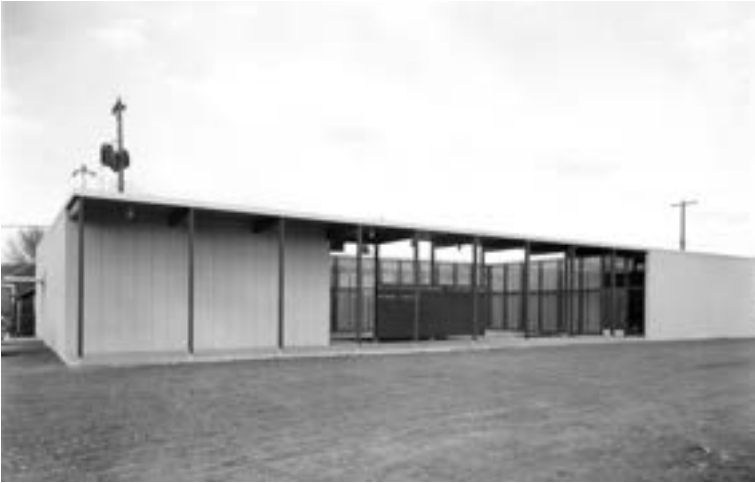
The original Inland Northwest AGC Building built in 1958.
