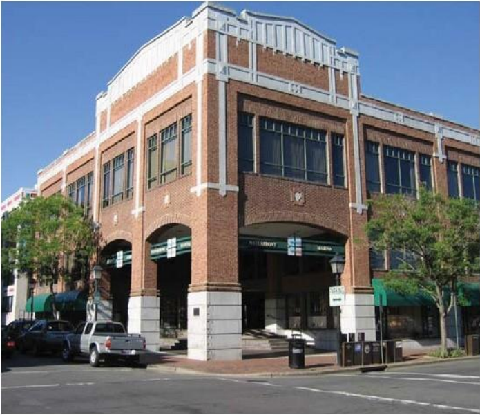
QUALITY REHABILITATION OF EXISTING BUILDING FACADE FACADE
