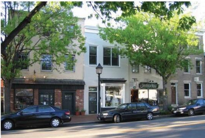
EXAMPLE OF WELL ARTICULATED FACADE AT STREET LEVEL
