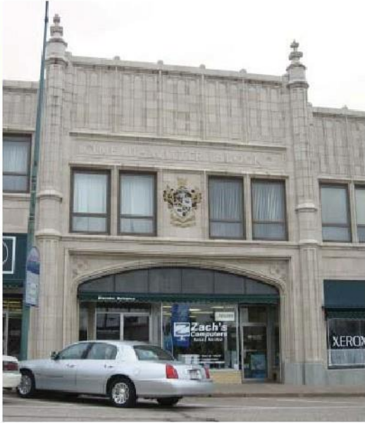
QUALITY EXISTING BUILDING
