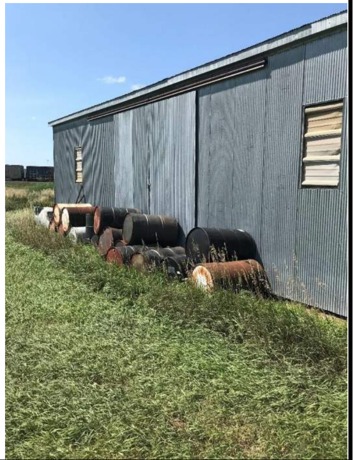
PHOTO 18: View of the empty 55-gallon drums located next to the southern storage outbuilding.
