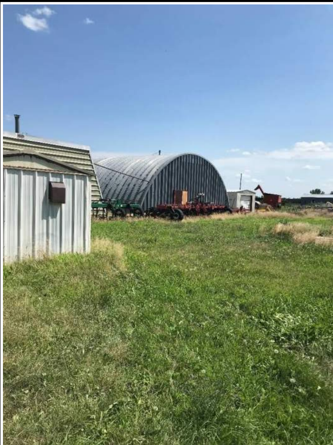
PHOTO 3: View of the Property from the northwest, looking southeast.
