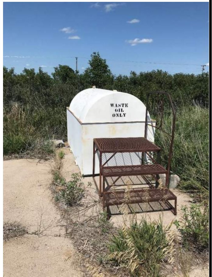
PHOTO 10: View of the 500-gallon waste oil AST located on the northern portion of the Property.
