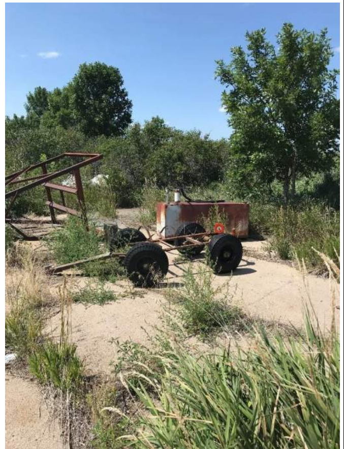
PHOTO 12: View of the empty 200-gallon AST located on the northern portion of the Property.
