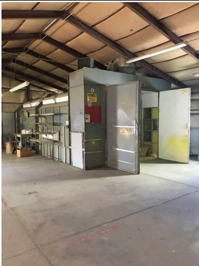
PHOTO 17: View of the paint chamber no longer in use.
