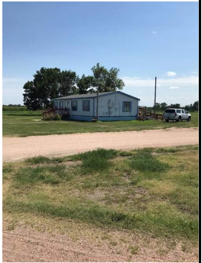
PHOTO 2: View of the Property from the north, looking southeast.
