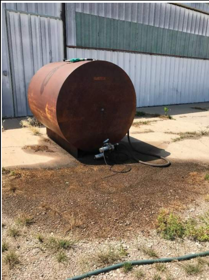
PHOTO 13: View of the 500-gallon diesel AST with staining located east of the northern shop building.
