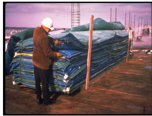
Protective blankets for curing in cold weather
