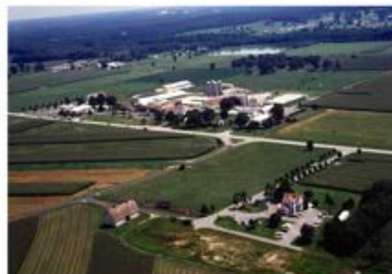
Aerial view of BARC Source: Ken Hammond - USDA ARS
