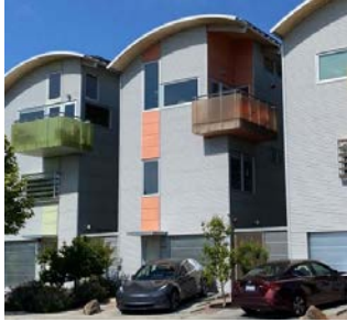
Figure 4.9 Example of what can happen without height standards calibrated to the existing context. These townhouses are “slot homes” that are out of scale with the existing context in terms of building height. They also fail to provide open space between units, making these less attractive to the consumer.
