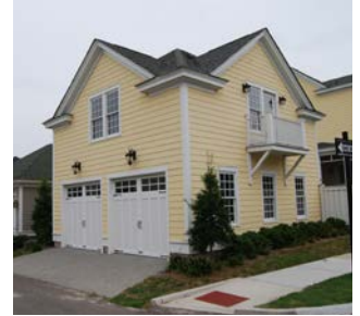
Figure 4.12 Example of an ADU used as either a guest suite, rental unit, or workshop/office over a garage.
