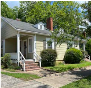
Figure 1.1 An example of a duplex MMH type with separate entries in Rock Hill.
