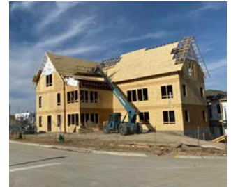
Figure 2.5 The simple forms, smaller size, and compatibility with simple wood-frame construction help maximize affordability and investment returns, and are consistent with the construction strategies familiar to most residential homebuilders, as shown in this under-construction MMH project in Papillion, Nebraska.
