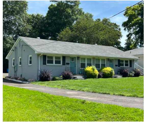
Duplex 2 units - Fort Mill
