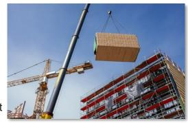
All loads also need to be inspected prior to lifting to ensure that all left behind items have been removed. such as lumber, wrapping bands, tools and debris. These items can easily be forgotten and become dropped objects.
