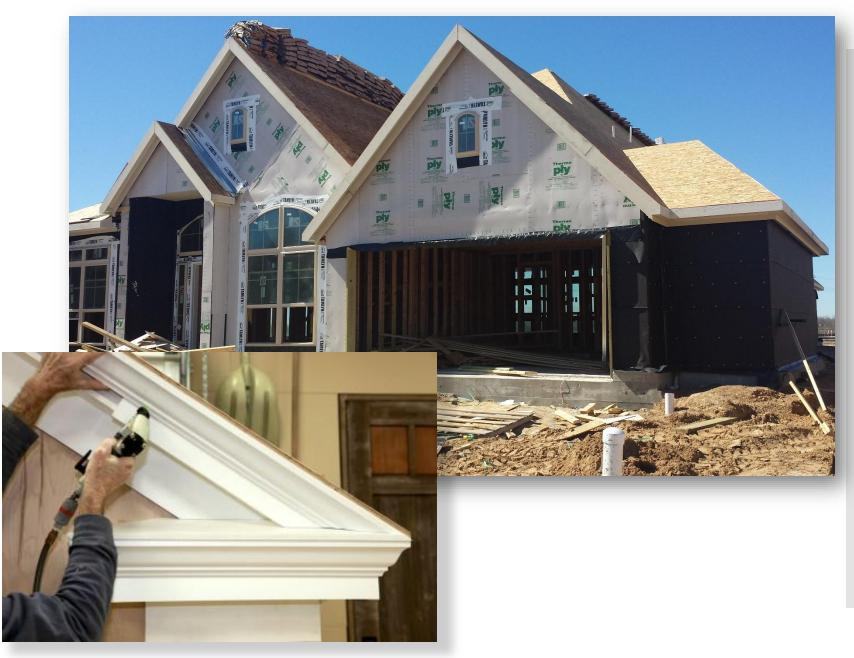
After the cornice stage the roof is decked with OSB (oriented strand board) to prepare it for shingles.
