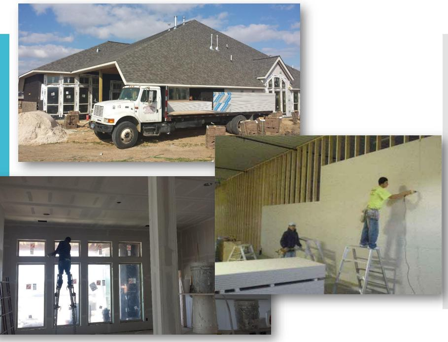
Sheetrock is a milestone because all of the mechanicals in the walls must be finished and insulation must pass a third party inspection.
