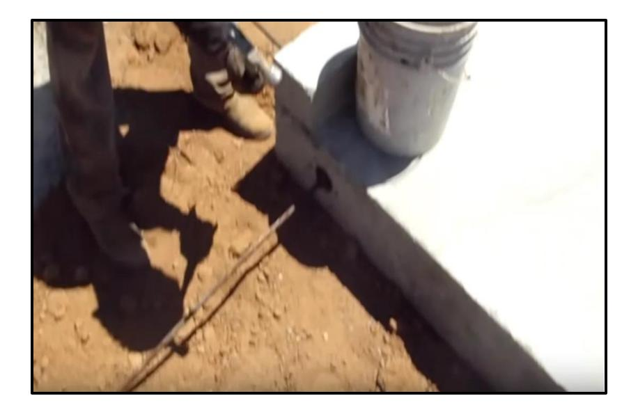
Pulling or stressing the steel cables squeezes the slab together preventing cracks in the foundation.
