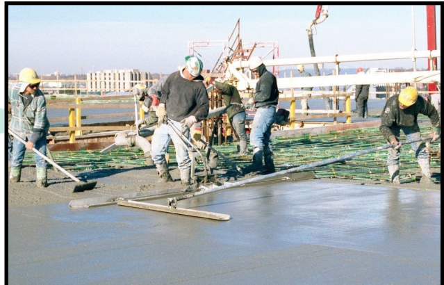
Construction Crew Finishing Concrete
