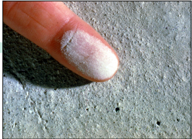
Dusting concrete surface
