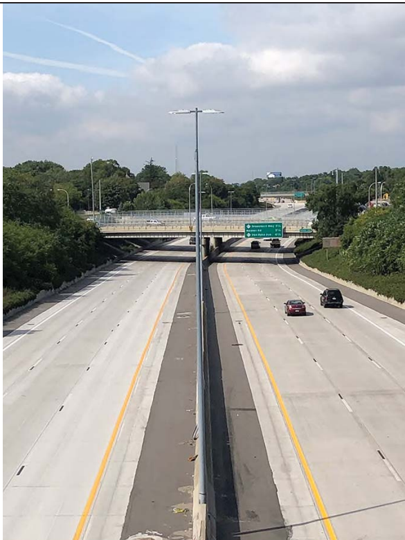
Photo 4 I-696 Completed Project Looking West Towards M-3 (Gratiot)
