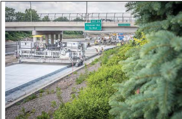
Photo 1 I-696 Paving of Concrete Inlay
