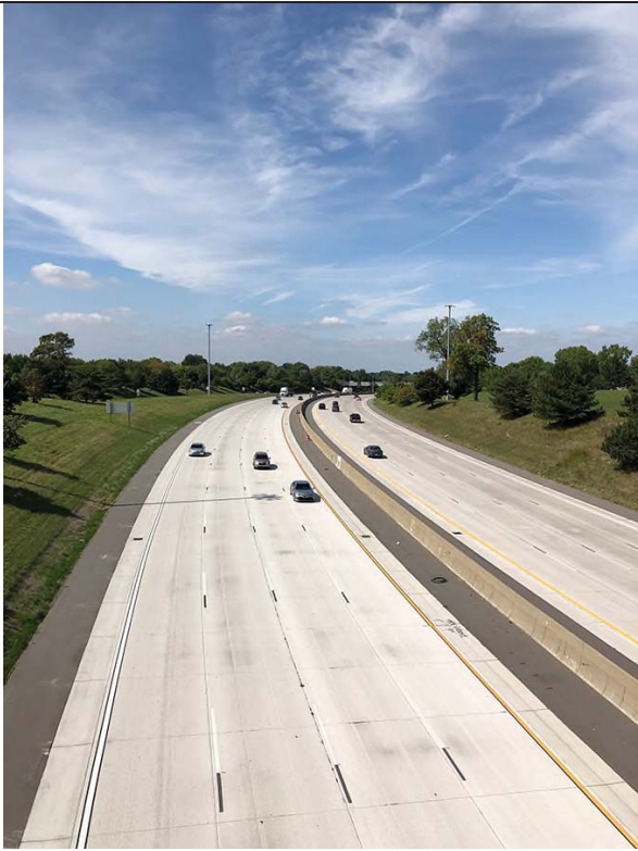
Photo 6 I-696 Completed Project West of the Mound Road Interchange
