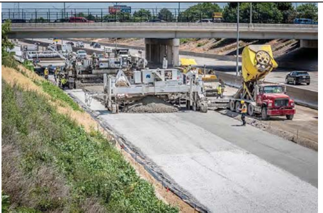
Photo 2 Paving of Concrete Inlay over Cement Treated Open Graded Drainage Course
