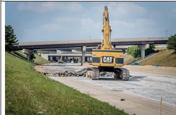
Photo 3 Pavement Removal Operation Near the Mound Road Interchange
