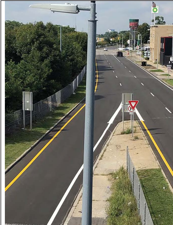
Photo 5 I-696 WB Service Drive and Entrance Ramp
