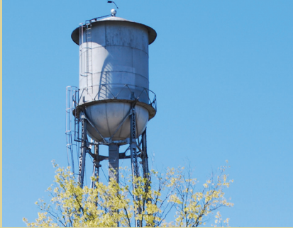
2. 134 JANESVILLE ST. Water Tower
