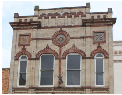
9. 117 SOUTH MAIN ST. Marvin Hardware/ Masonic (1898)
