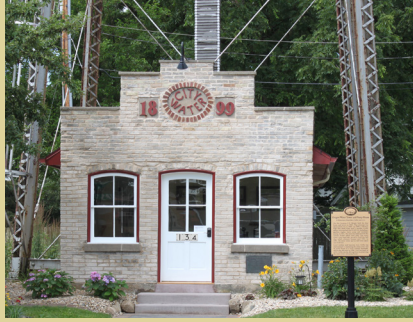
1. 134 JANESVILLE ST. Welcome Center - Pump House
