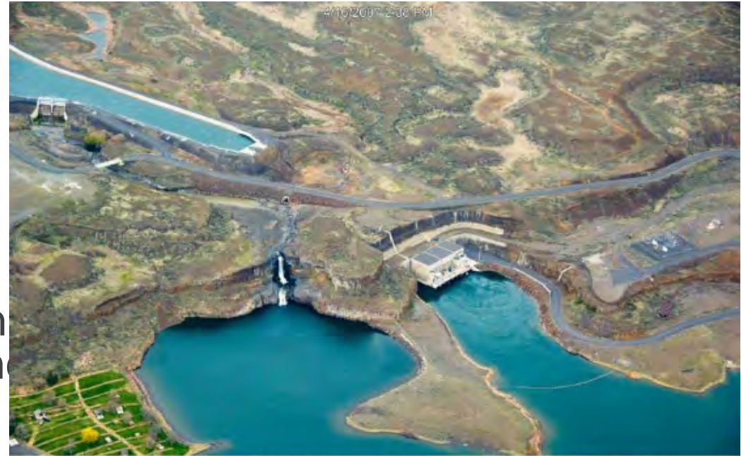
Billy Clapp Lake, Summer Falls & Columbia Basin Project Main Canal (4/16/2007)
