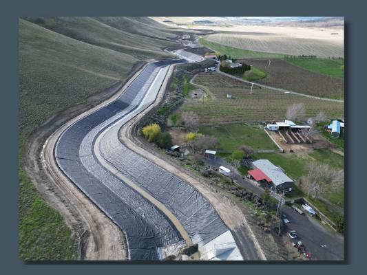
**Material** Lined with 60mL thick High-Density Polyethylene (HDPE) Liner which is thicker than typical buried liners, to account for UV degradation over time.
