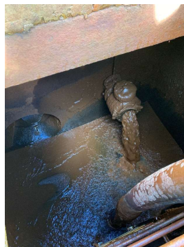
Sludge Blowdown Discharge into the East Chamber
