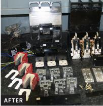
After initial inspection and apparatus testing, PEARL Reconditioning standards require full disassembly as part of the reconditioning process. After all parts have been cleaned, reconditioned — and when necessary — replaced, the device is tested again to make sure it meets minimum performance specifications as set out by the OEM when the apparatus was first manufactured.
