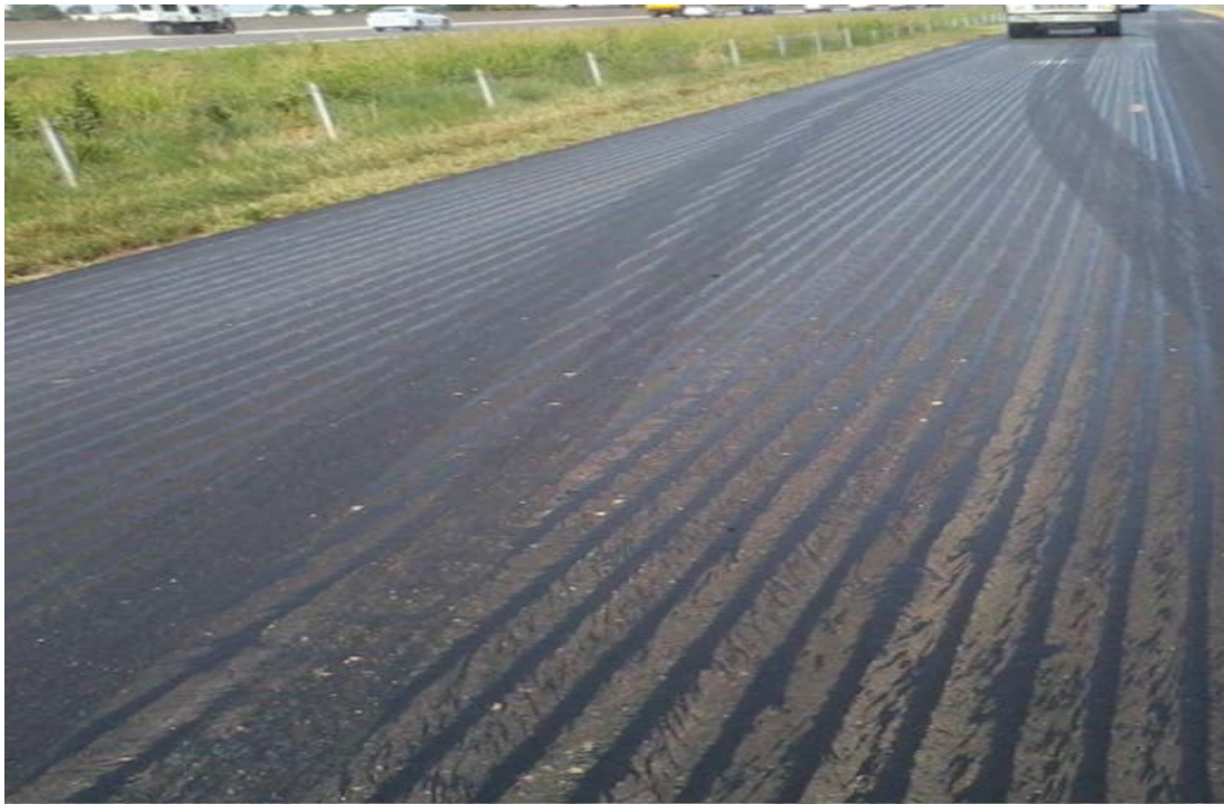
Figure 5. A uniform tack application.
