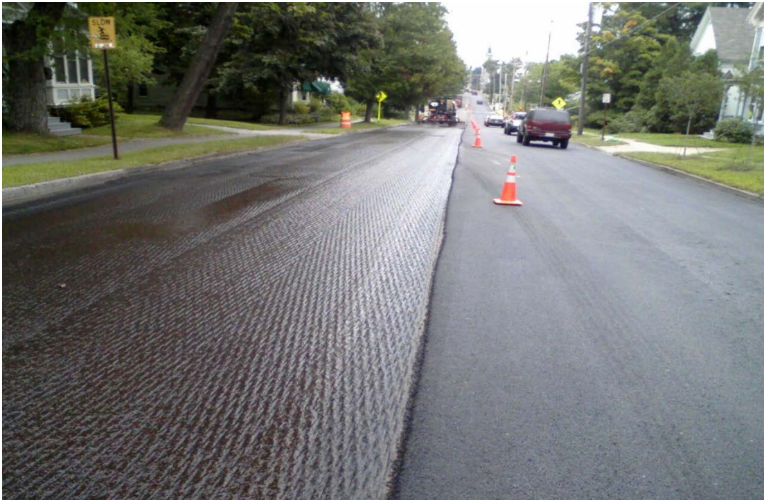
Figure 5. A uniform tack application.
