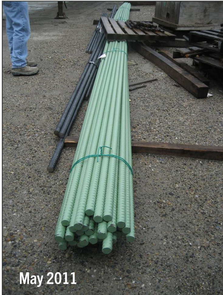
Bundle of PT bars in precast yard
