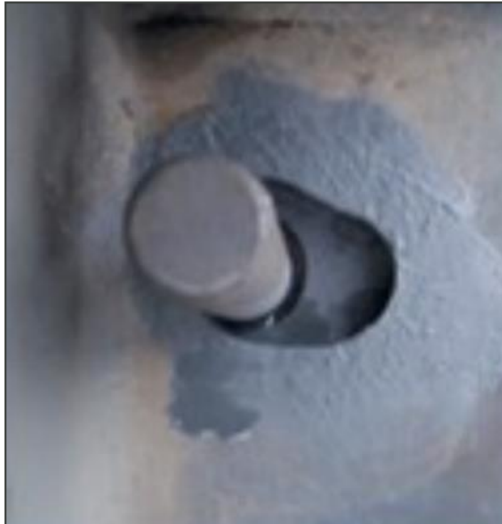
Modified 1-1/8 in. Diameter Anchor Rods Connection
