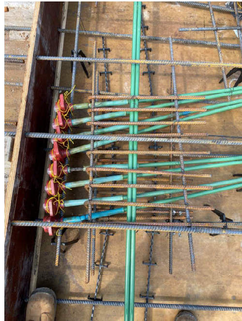
Fig. A6—Two-way slab system exterior columns. (Note: 1 in. = 25.4 mm.)
