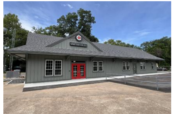
Smithville Station completed
