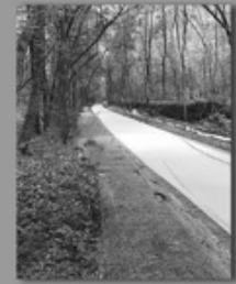
STABILIZED STONEDUST® TRUNKLINE TRAIL
