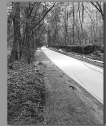
STABILIZED STONEDUST® TRUNKLINE TRAIL
