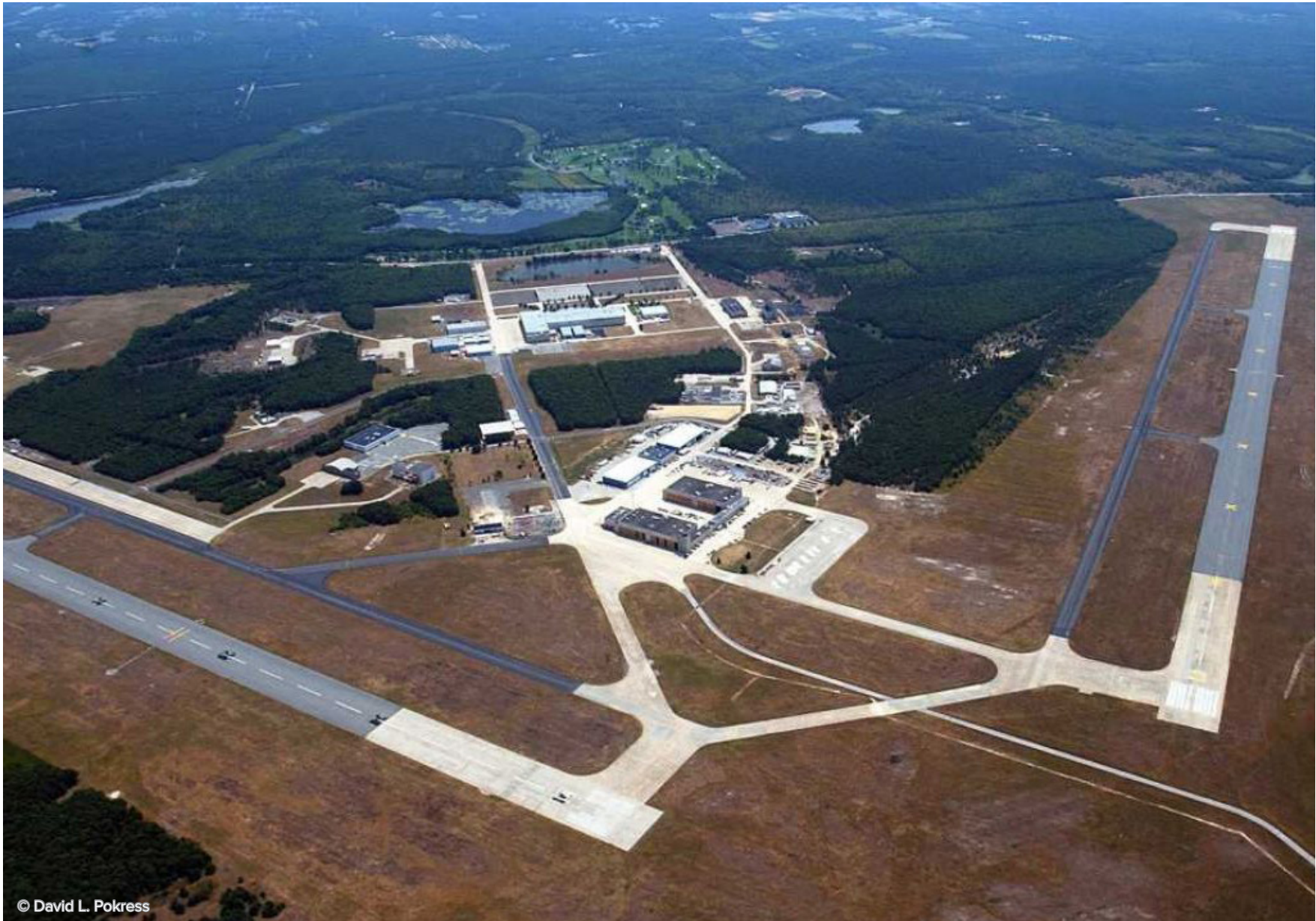
Figure IV-5: The Calverton site
