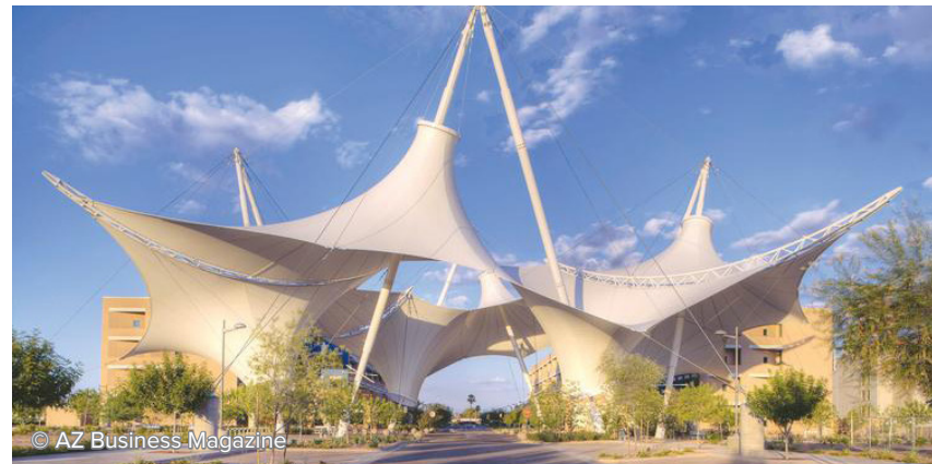
Figure V-3: SkySong's public plaza and tensile structure - an example of public realm improvement
