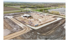
Clay County Jail & Law Enforcement Center Under Construction
