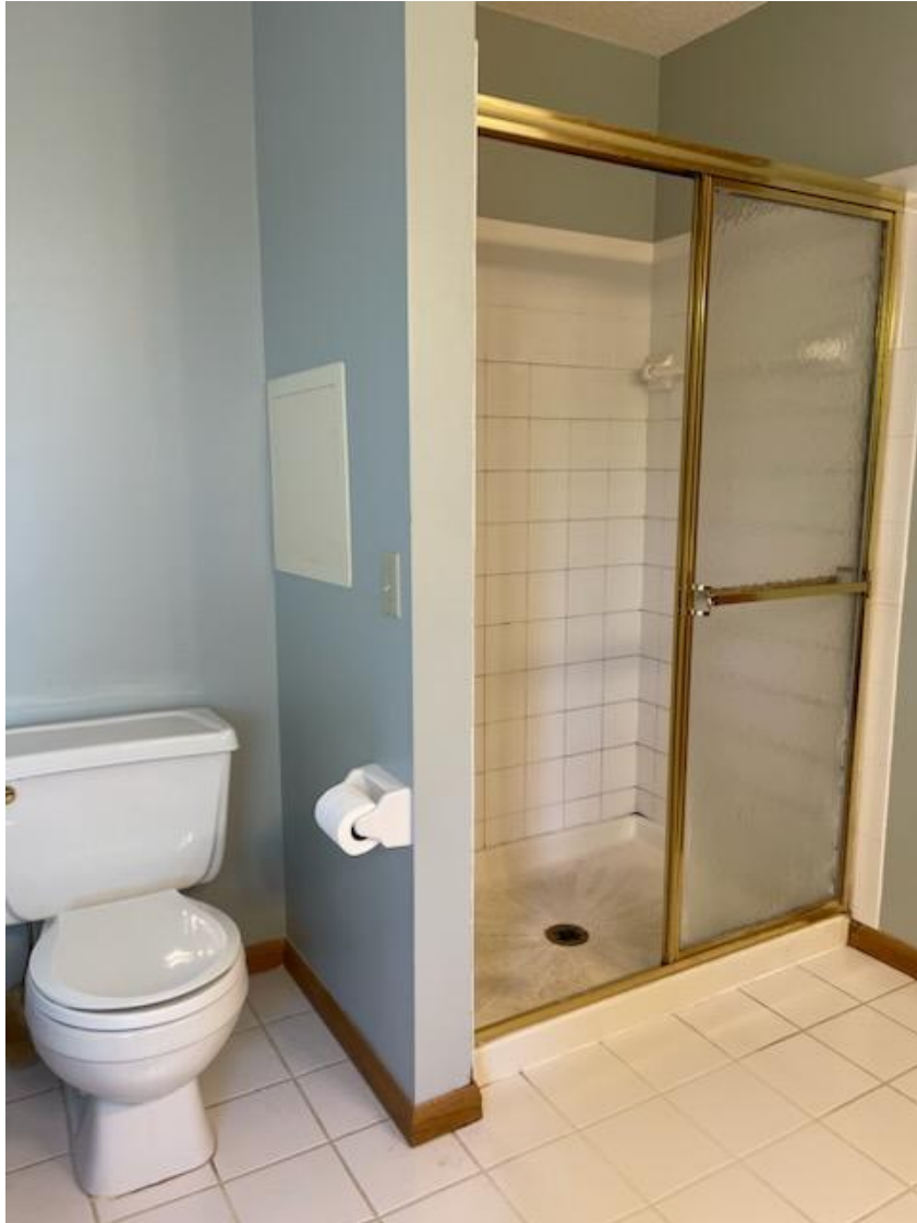
The curbed shower was worn and dated.
