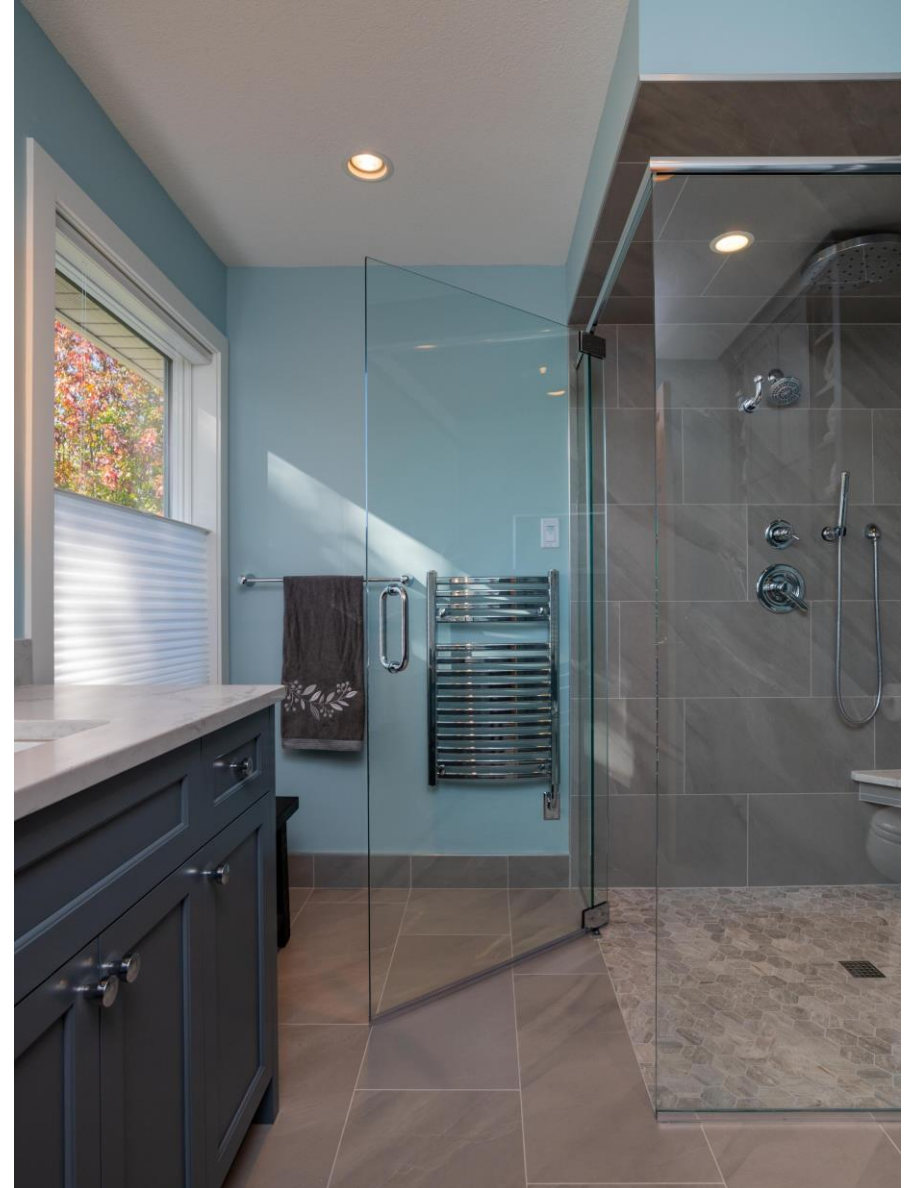
The shower was moved. Frameless glass shower walls and door (swings both ways) give an open, airy feel to the space.
