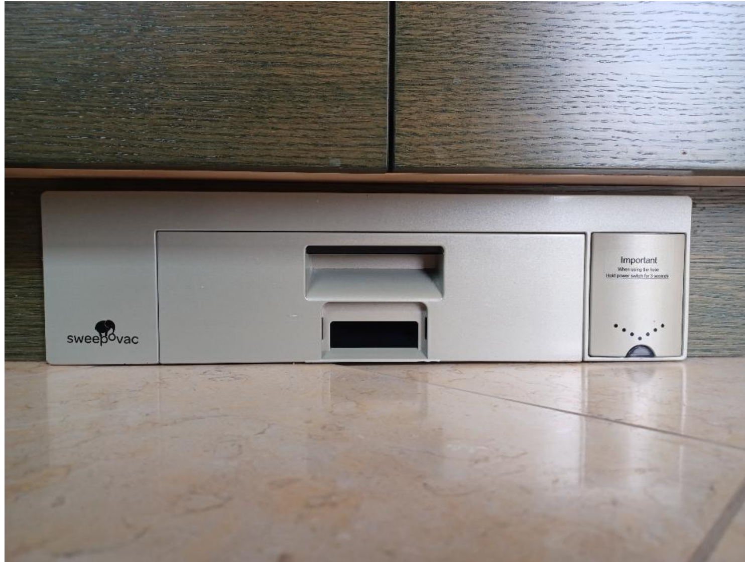
Sweepovac Big Kick, a space-saving, concealed powerful vacuum was installed. Kick the button on the right and kitchen floor debris is quickly extracted.
