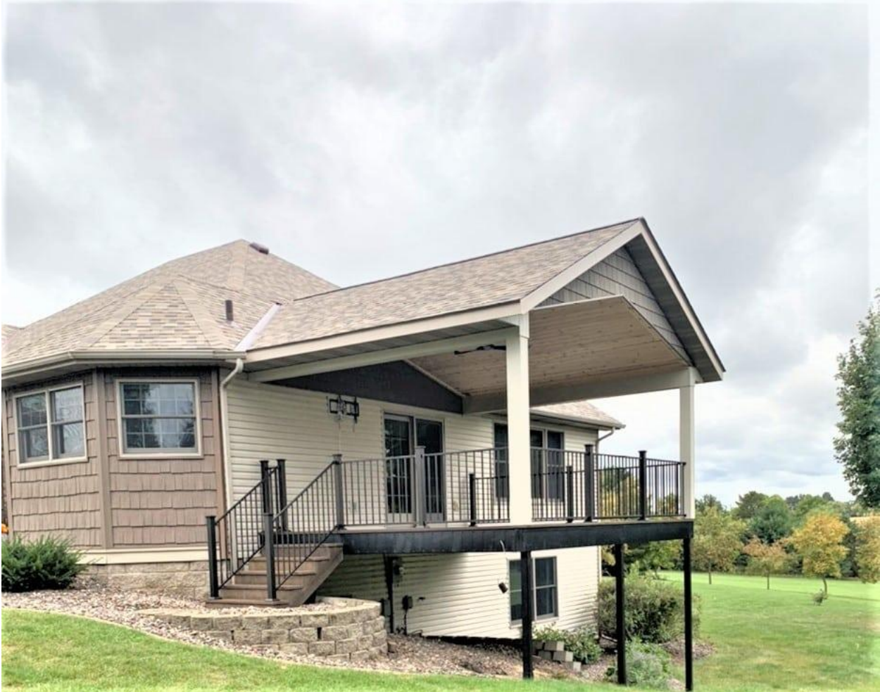
Photos showing the completed project
