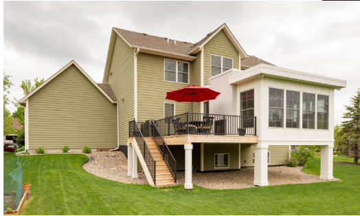
Residential Addition $100,000 to $250,000 AMEK, Inc. - SILVER
