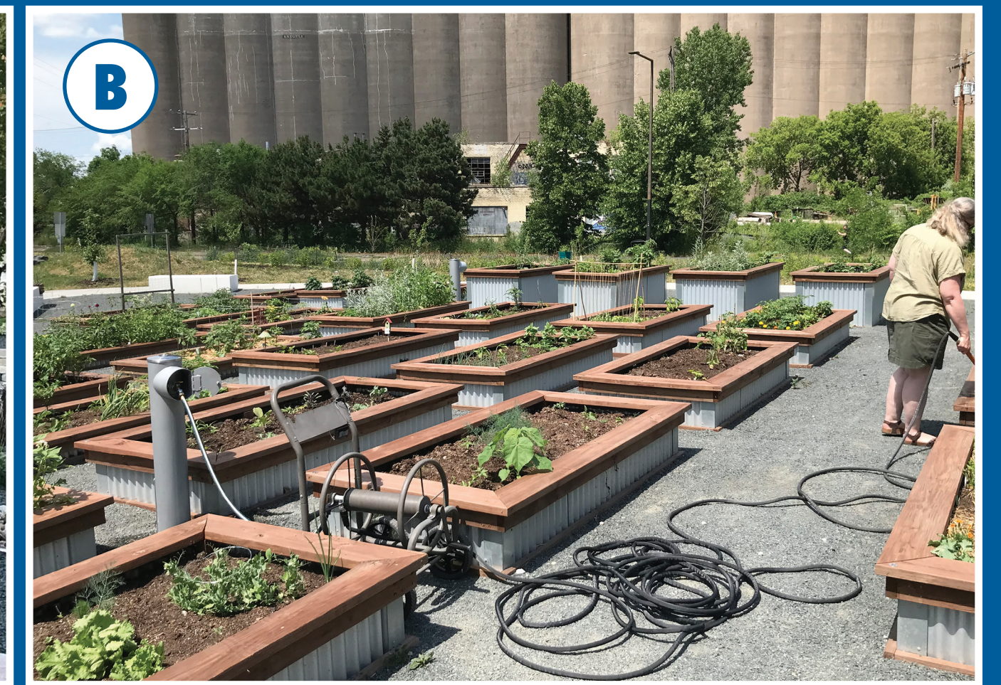
B Drought-tested, the stormwater reuse system distributes over 100,000 gallons of irrigation water. UV treatment allows for community garden use, possibly a first in Minnesota.
