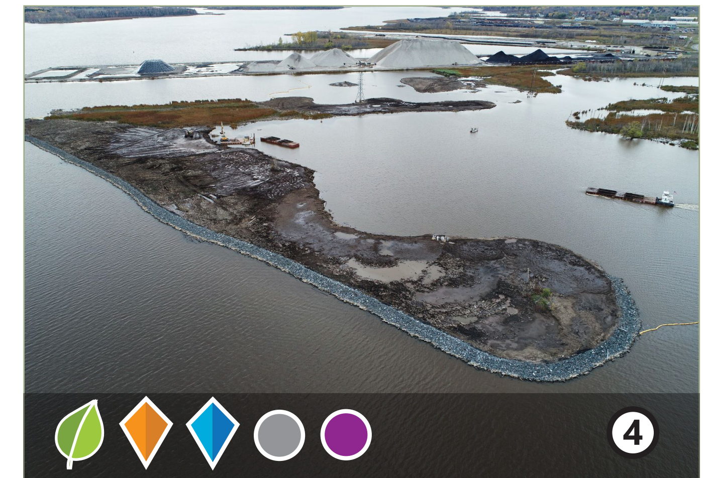
Existing island built up and extended to create a shallow, sheltered bay setting
