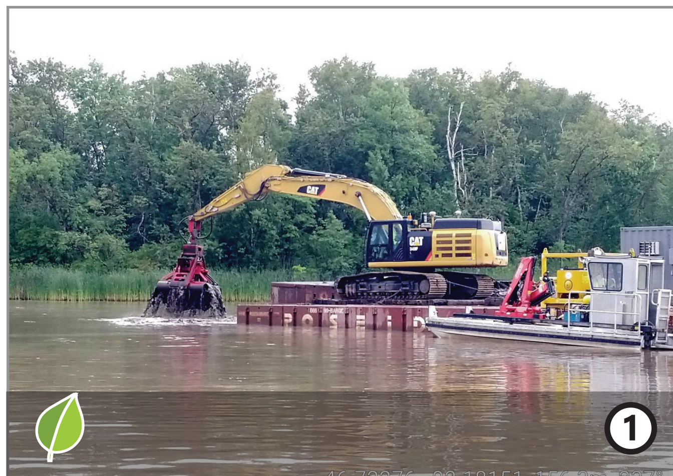
Removed invasive species community and dredged nuisance sediment to deepen bay
