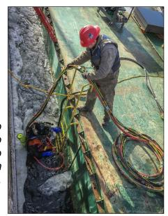
A diver is lowered into the lock chamber to conduct guidewall crib repairs at Lock & Dam 8 in Genoa, Wisconsin, on Jan. 9, 2018.
