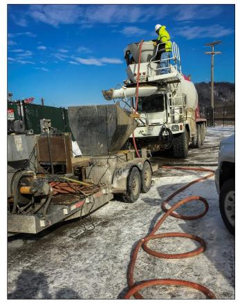
Crews prepare the concrete while conducting guidewall crib repairs at Lock & Dam 8 in Genoa, Wis., on Jan. 17.
