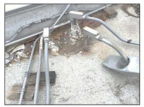
roof, an equipment grounding conductor of the wire type shall be installed in outdoor portions of metallic raceway systems that use non-threaded fittings.
