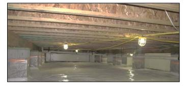
(E) Crawl Space Lighting Outlets. GFCI protection shall be provided for lighting outlets not exceeding <u>120 volts installed in crawl spaces</u>. Fatal incidents have shown amp guards do not provide appropriate shock protection. The GFCI requirement applies to lighting outlets in both dwellings and non-dwellings.
