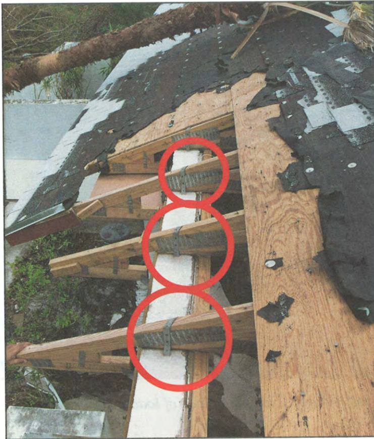
FIGURE 56. Properly placed hurricane straps from masonry tie-beams to roof trusses.
