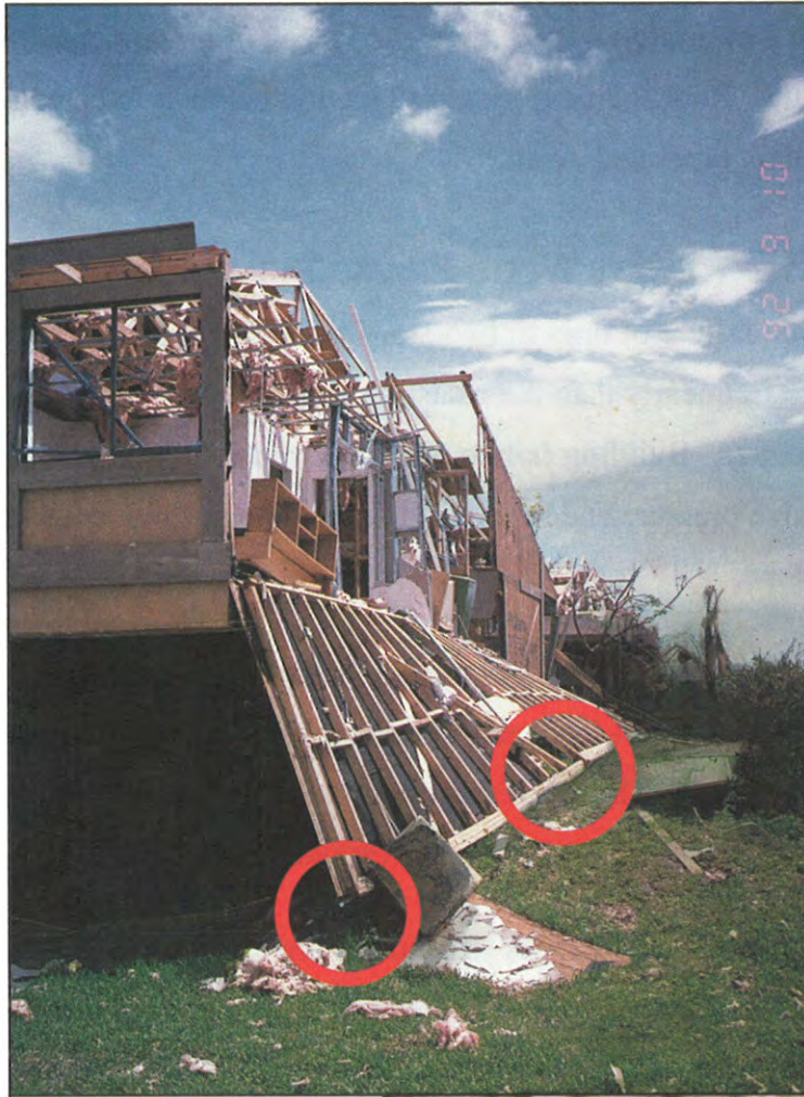
FIGURE 4. Exterior wood-frame non-loadbearing wall. Transfer of wind forces from wall to adjoining structure was not sufficient.
