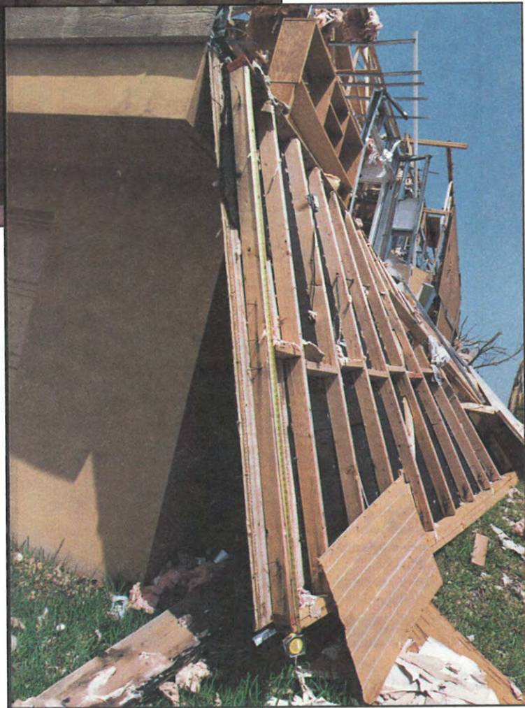
FIGURE 60. Side wall failure. Side wall has no lateral load transfer capacity due to inadequately built-up corner post.
