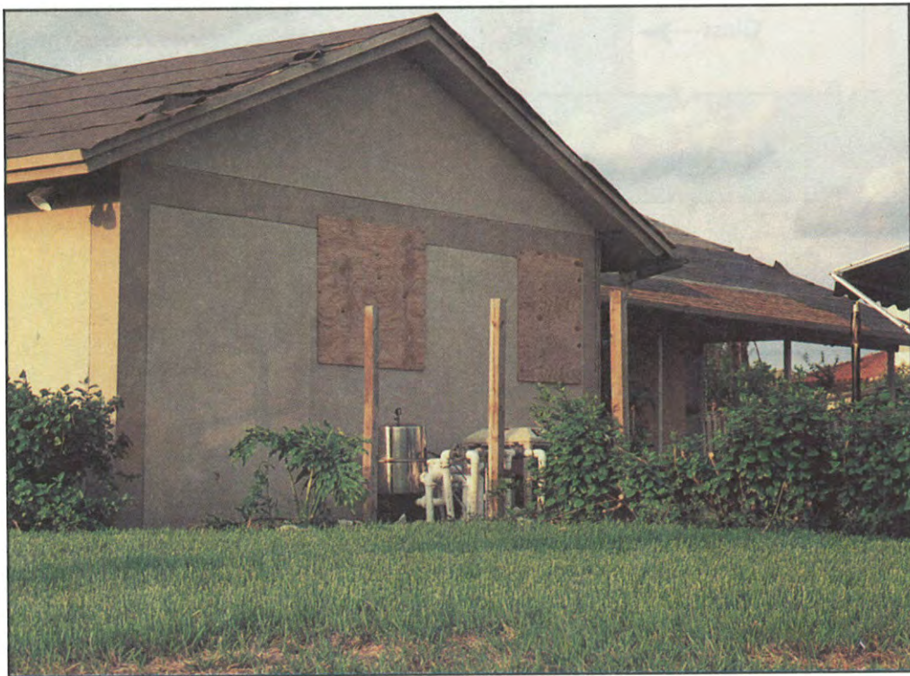
FIGURE 51. Plywood used as openings protection installed. See Figures 52 and 53 for details.
