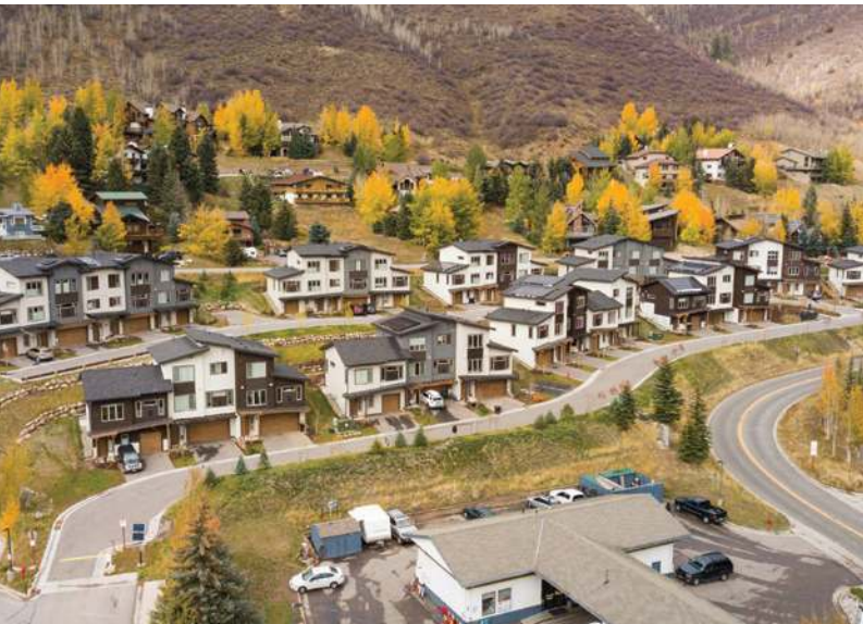
Townhouses in Vail, CO from Prefab Logic and DCI Engineers
