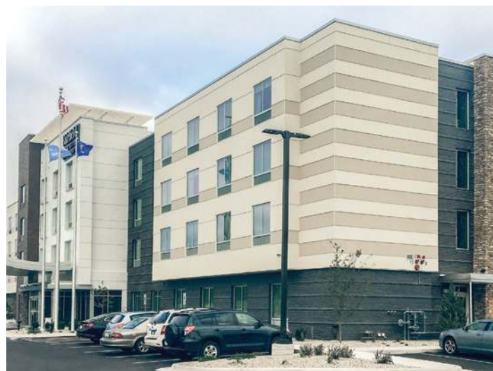
Fairfield Inn & Suites in Pleasant Prairie, WI from Champion Commercial Structures and Hayes Modular.
