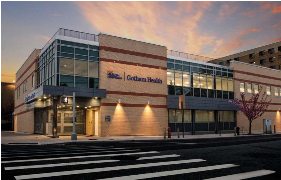
Gotham Health – Vanderbilt Family Health Clinic in Staten Island, NY from Axis Construction Corp. and NRB, Inc.
