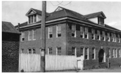
The historic appearance of the Jefferson School circa 1940-1950
