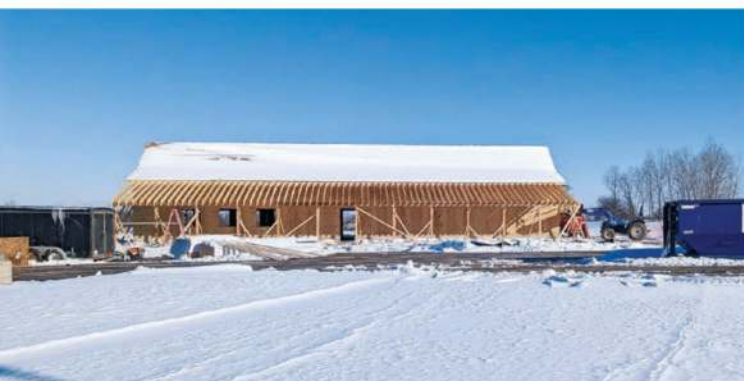
Under Construction: Ottawa + Allegan On the Ridge.
