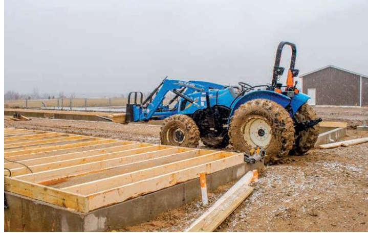
Under Construction: Ottawa + Allegan On the Ridge.
