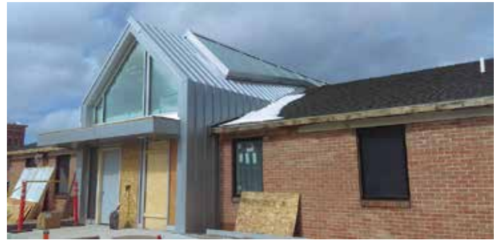
Metal roof installation at south entrance.
