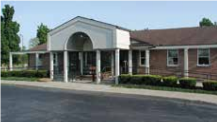
Chamber building before.
