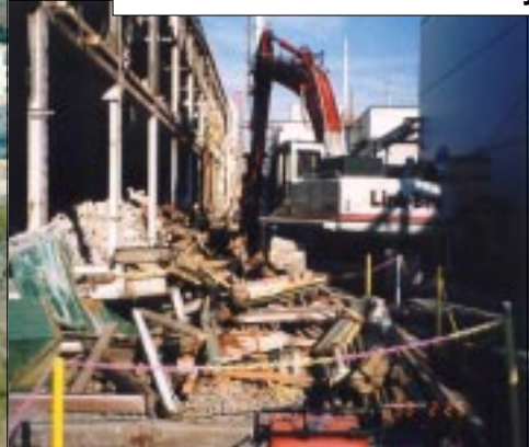
K-1131 Demolition Under Way
