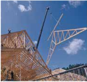
Roof & Floor Trusses
