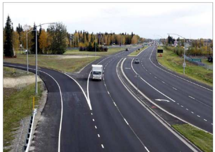
Fairbanks Airport Way Repaving Phase 2, HC Contractors, Inc.
