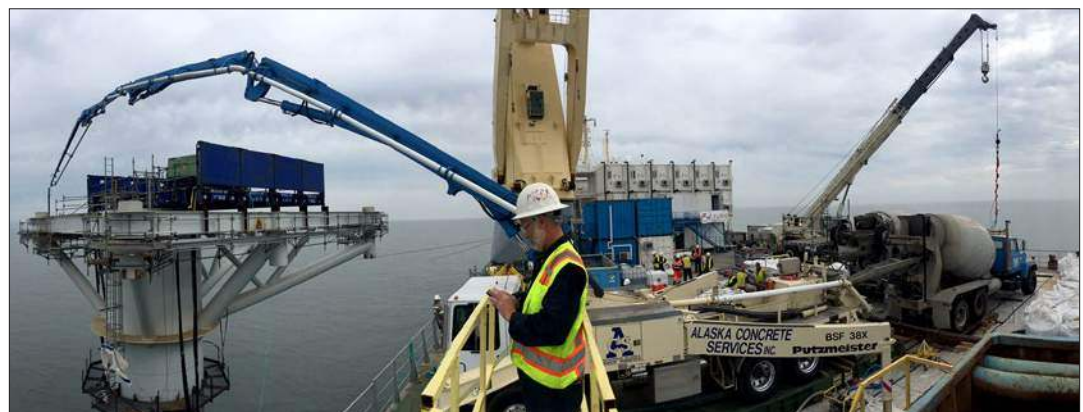
KLU#3 Furie Platform Grout Seal Remedial Work, Davis Block Co., Inc.
