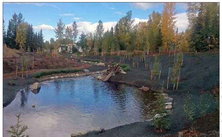
Chester Creek At Muldoon Realignment, Anchorage, Bristol Construction Services
