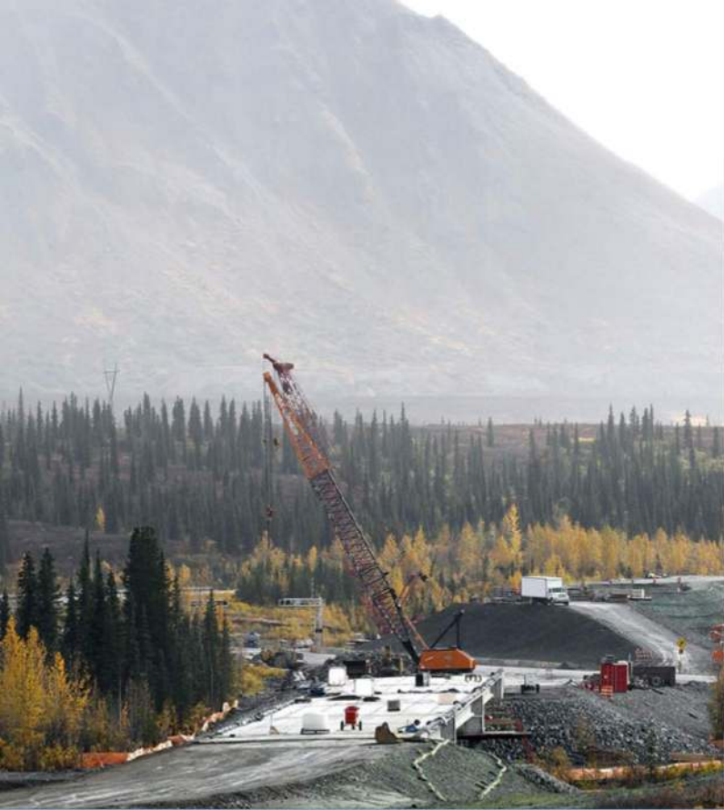
Middle Fork Chulitna River Bridge, Quality Asphalt Paving (QAP)
