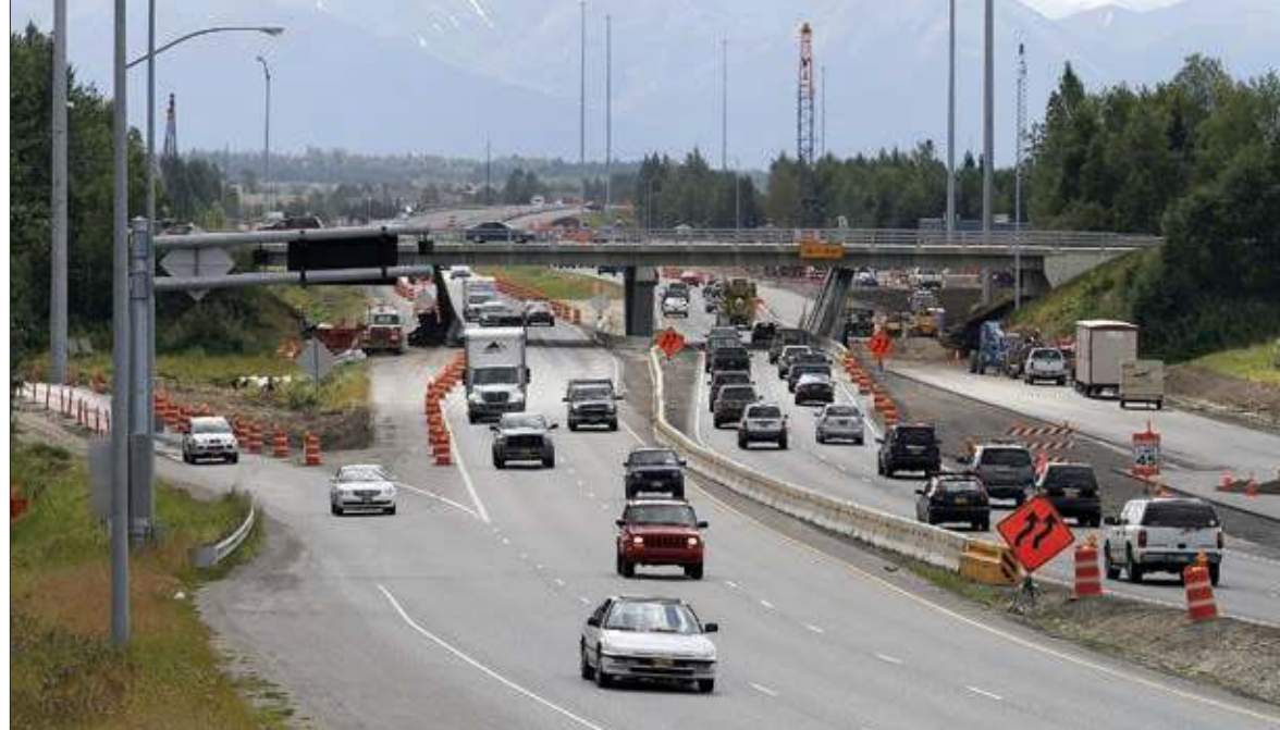
Seward Highway Improvement, Anchorage, QAP
