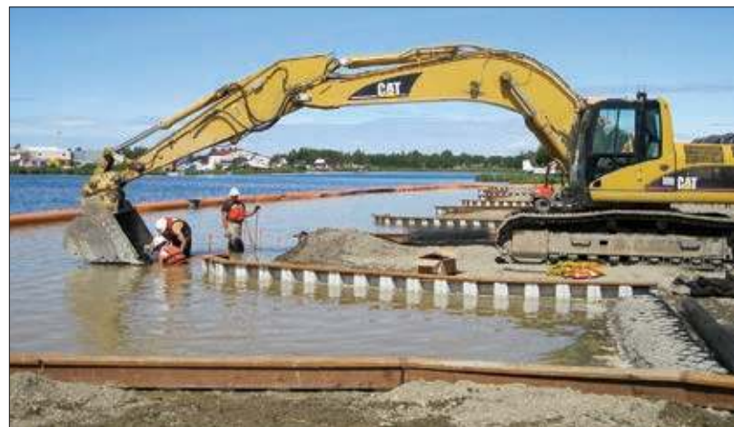
Lake Hood Bank Stabilization, Anchorage, Granite Construction
