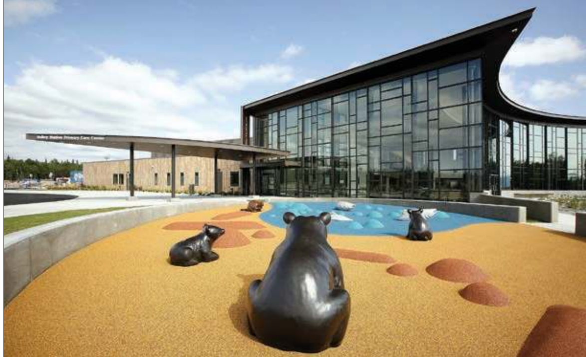
Valley Primary Care, Wasilla, Neeser Construction
